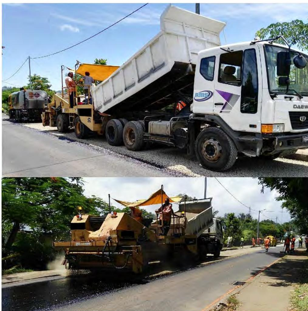
Urban Roads and Drainage Phase 1 contractor, RMS, and sub-contractor Downer, began road sealing in January. The project will seal 13 km of Port Vila roads with a double coat of rubberized bitumen seal (hot tar). This waterproof coating
